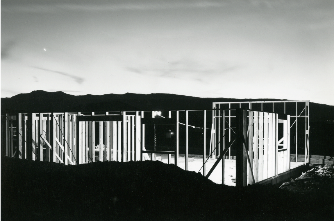
Night Construction, Reno, 1977
