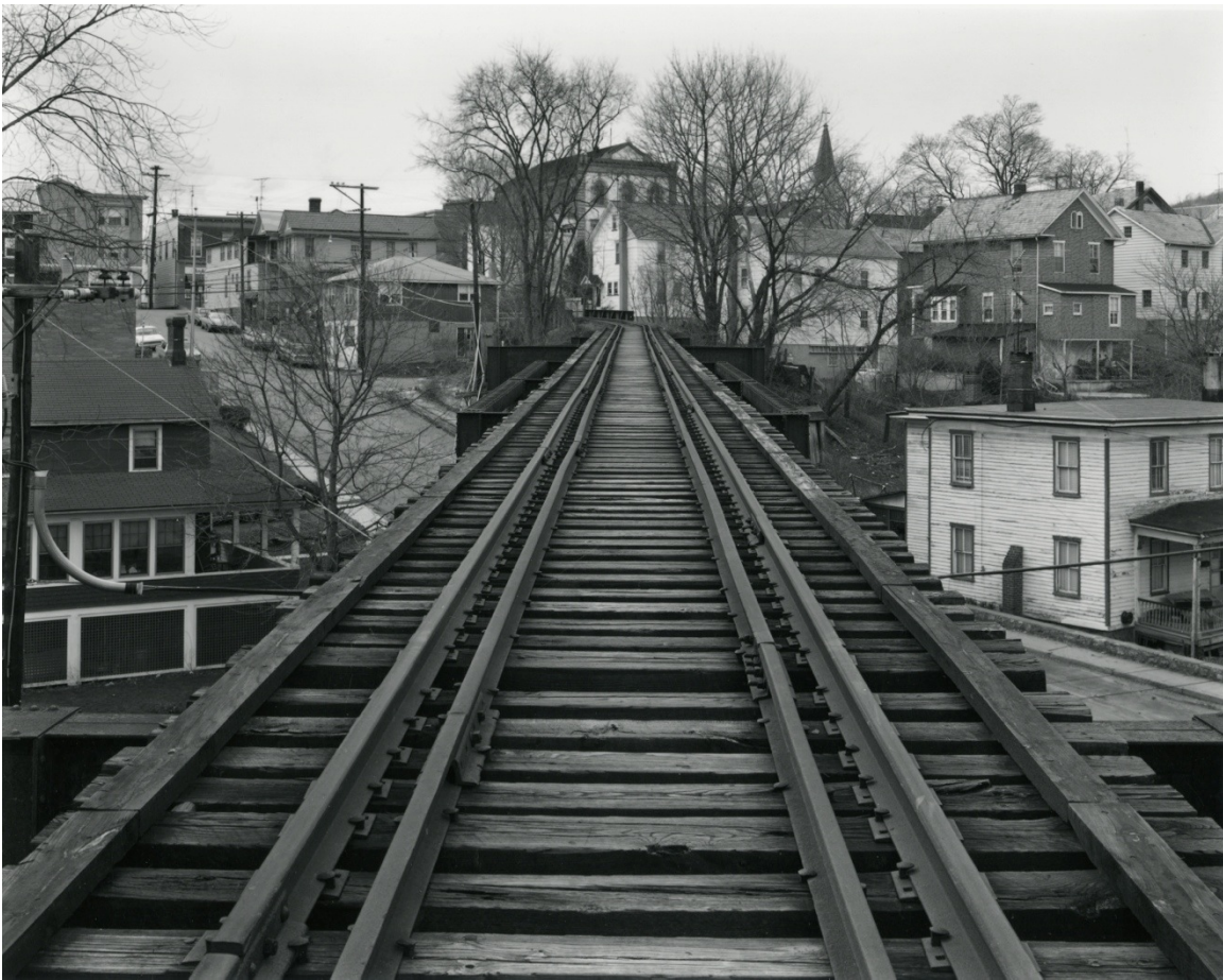
Railroad Bridge, High Bridge, NJ. 1974
